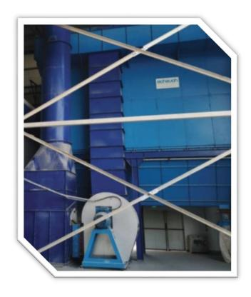
It is intended for removing of white fumes containing zinc dust particles from area above zinc melt and it consists of exhausting pipes, filter with air pressure regeneration and fan.
